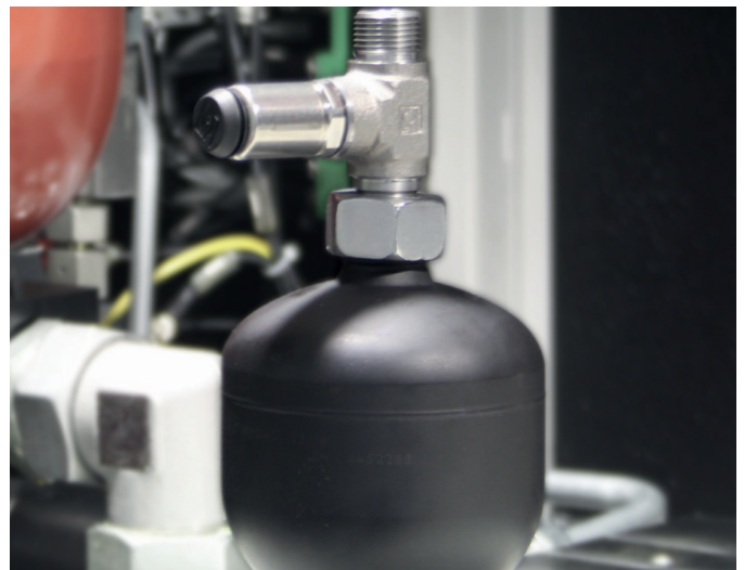
Diaphragm Accumulator Adaptor
